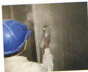
Grinding Concrete
