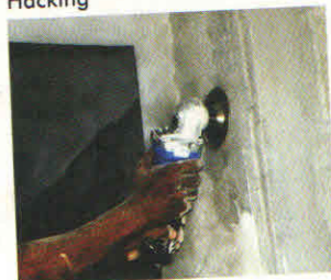
Removing Plaster
